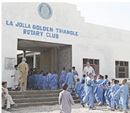
The Rotary Club of La Jolla Golden Triangle, California, USA, recently helped build a school in Jalalabad, Afghanistan.
